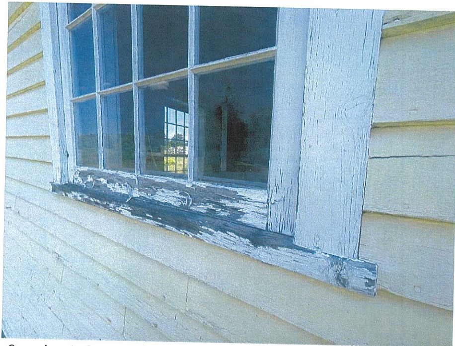
Sample window condition. Windows will be restored and repainted.
